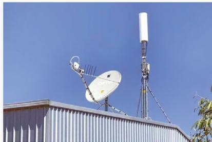
Optimized for satellite backhaul, Gilat’s CellEdge Small Cell Over Satellite backhaul solution delivers the same speed and quality as a terrestrial backhaul solution. CellEdge SDR uses the open standard luh interface, enabling satellite bandwidth optimization for high efficiency and data rates.
